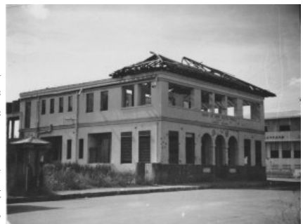
The damaged Bank of NSW in Darwin
