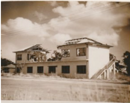
A damaged building in Darwin
